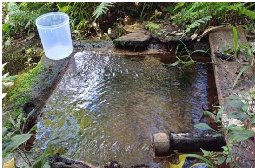
Figure 2. Condition of The Reservoir at Liubena Spring (Source: Researcher Documentation, 2023)
